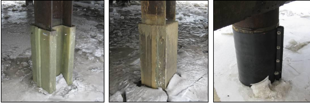
Figure 8. H-Shaped, Rectangular, and Pipe Pile Protective Systems
