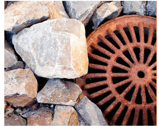
The Brewery, infiltration trench, Milwaukee
