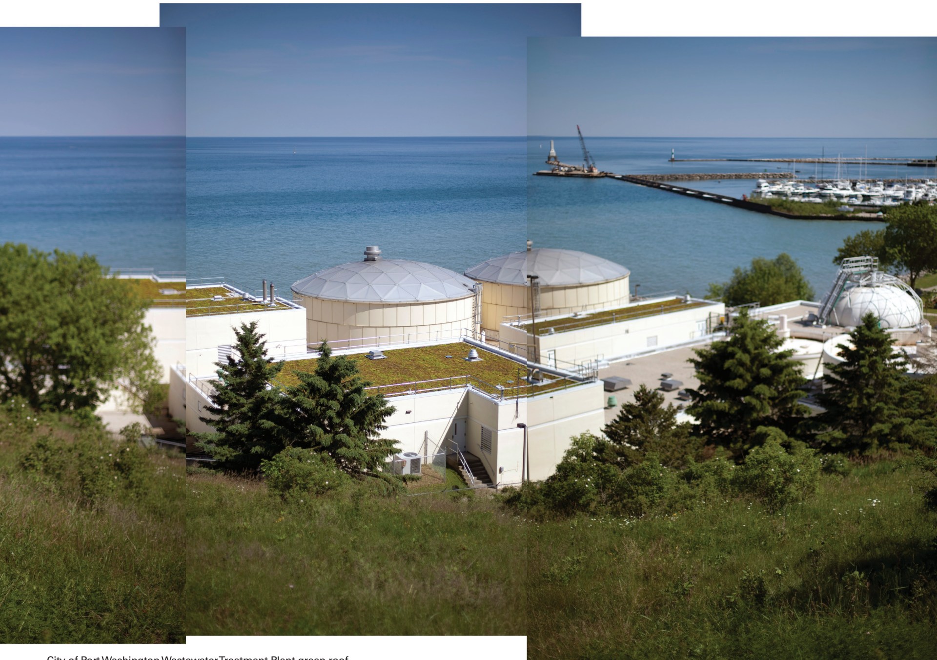
City of Port Washington Wastewater Treatment Plant green roof
